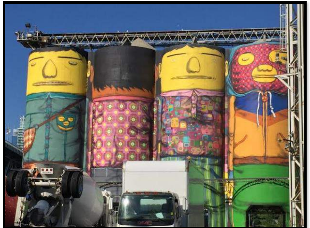
Photo: Silos in Vancouver, BC, Brent Toderian
