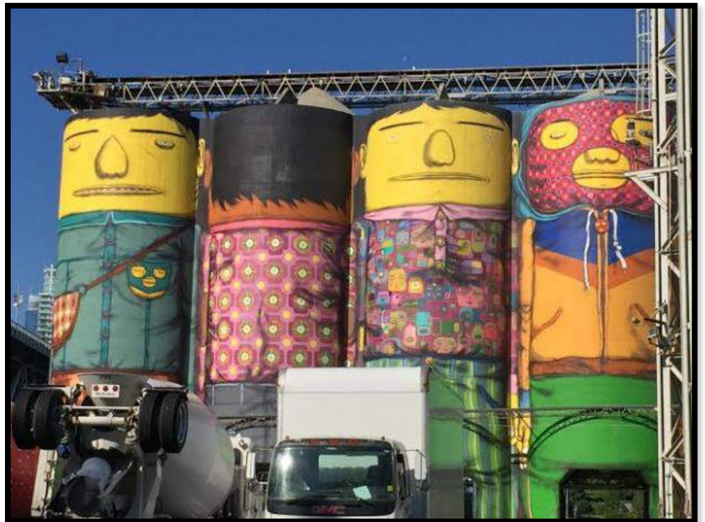
Photo: Silos in Vancouver, BC, Brent Toderian
