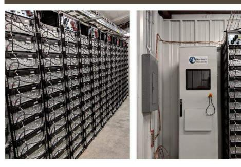
Racking Configuration is 13 x 2 and the top section is used for mounting Switchgear
